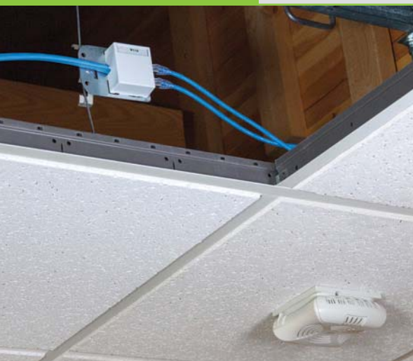
QuickPort® In-Ceiling Bracket with clip and Surface-Mount Box
